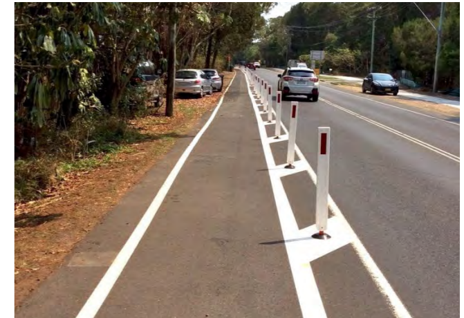
Broken Head Bike Path, Byron Shire (Image © Durapost)
