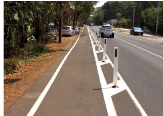
Broken Head Bike Path, Byron Shire (Image © Durapost)
