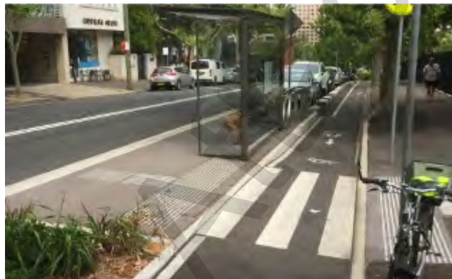
Figure 9: This design maximises safety for cyclists and bus passengers, by using the bus stop as a buffer between the bikeway and the road.
